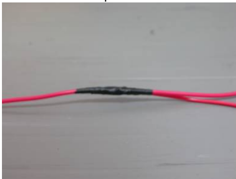
Figure 6: Isolate the Connection
