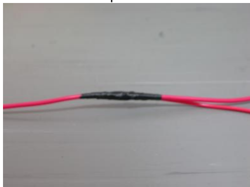
Figure 7: Isolate the Connection
